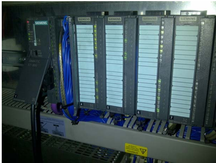
Figure 2.2.A PLC Rack
