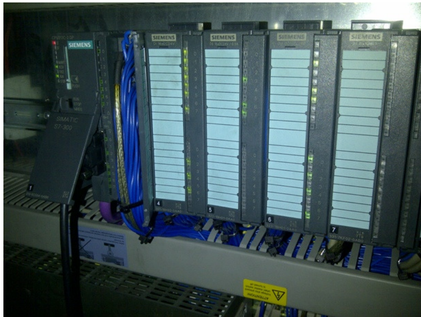
Figure 2.2.A PLC Rack
